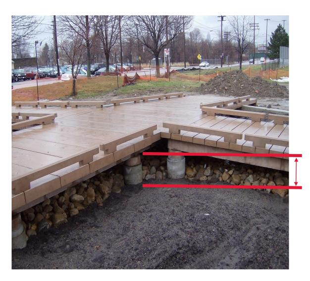
Less than 30"No Handrail Required
