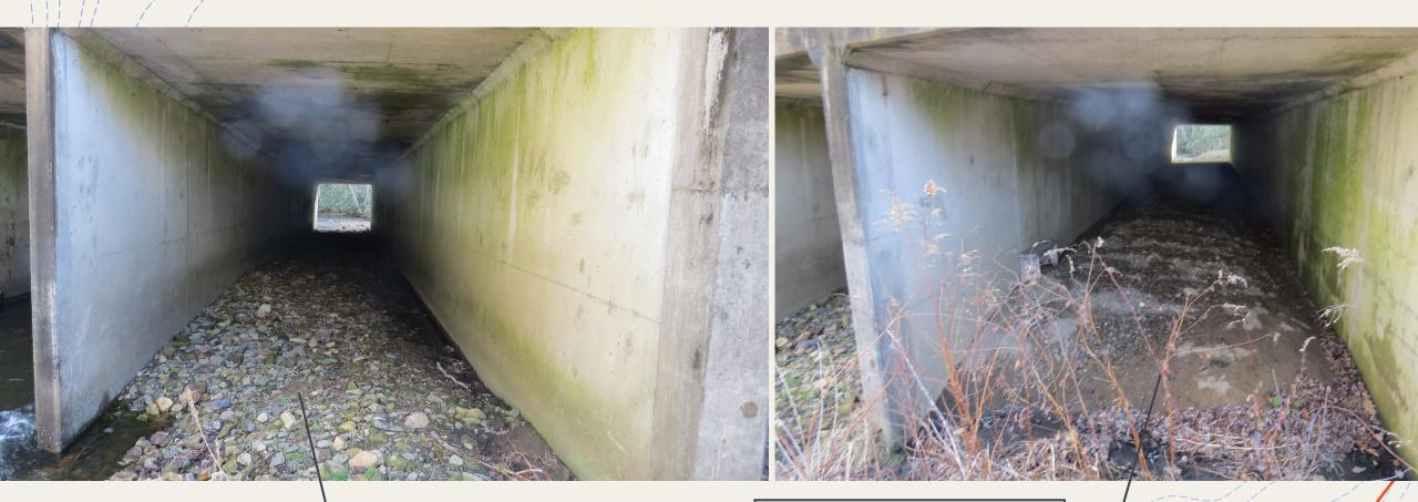
Middle Culvert – Note Cobble Sized Substrate
