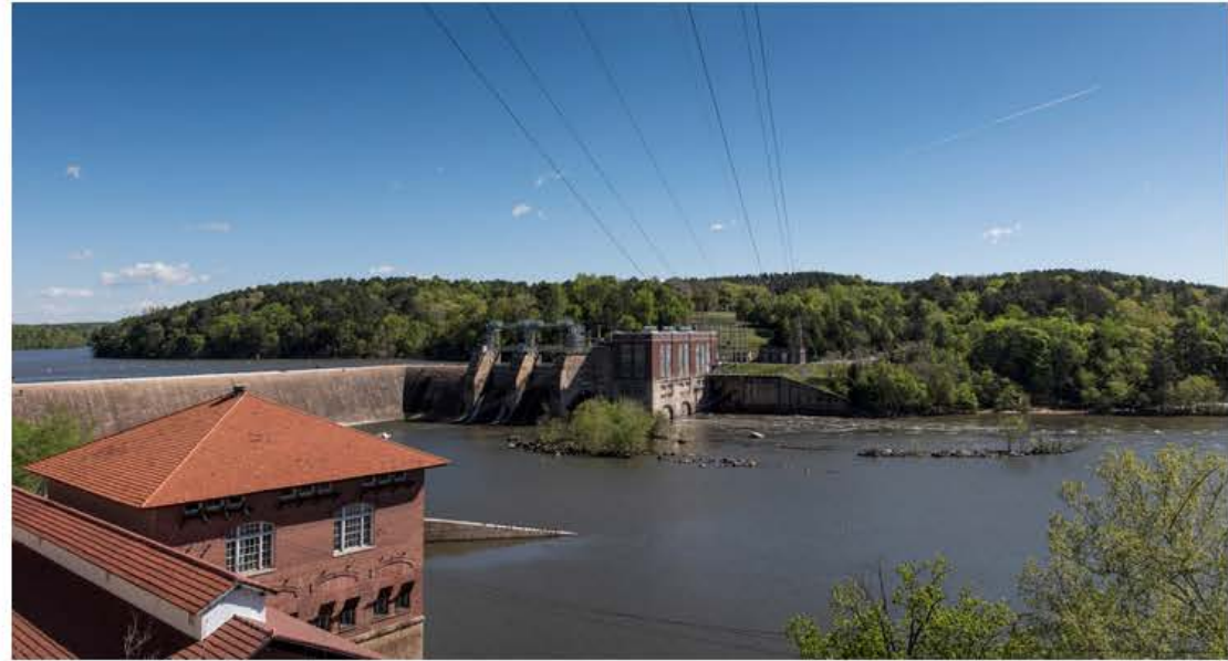
Rocky Creek hydroelectric plant, located just downriver from the future park (Image: Duke Energy)
