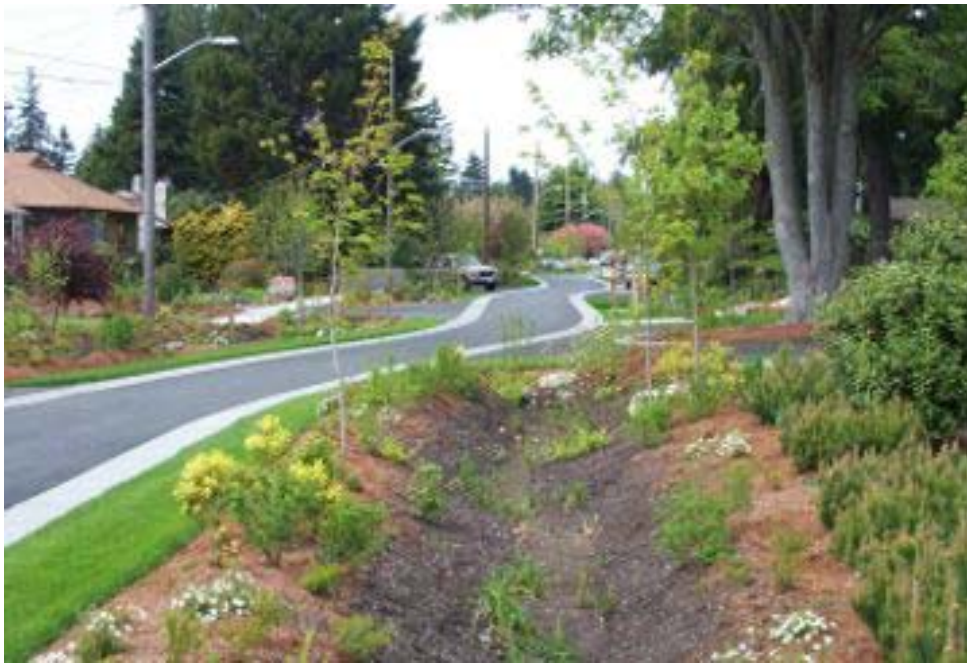
Image C.2: Roadside Swale
