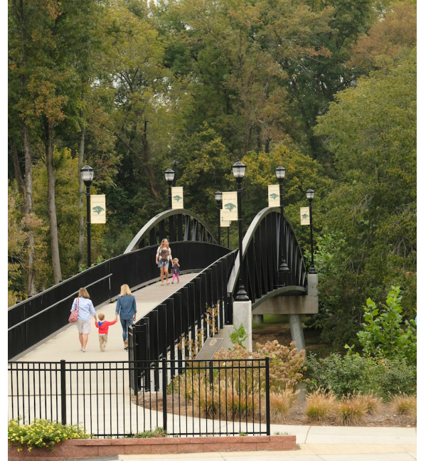
In 2015, a new pedestrian bridge spanning the South Fork River connected Goat Island Park to Cramerton's central business district. The bridge and the Goat Island Greenway are a major section of the Carolina Thread Trail in Gaston County. Photo by Nancy Pierce
