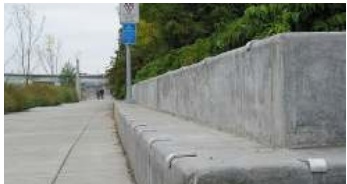
Retaining wall doubles as seating
