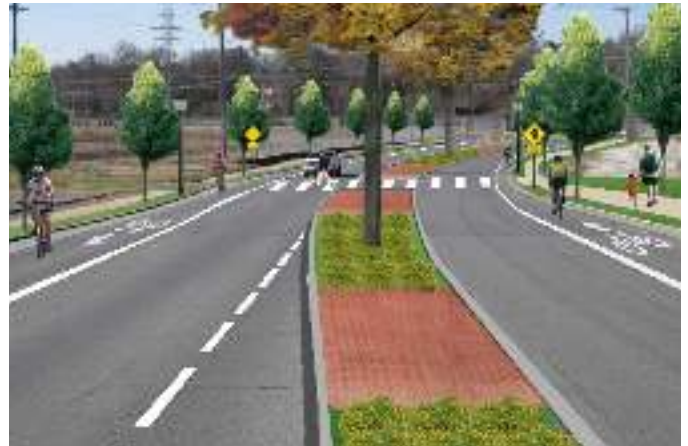
Old Salisbury Road with a median that also serves as a pedestrian refuge island. Refuge islands reduce the time pedestrians are exposed to vehicular traffic.
