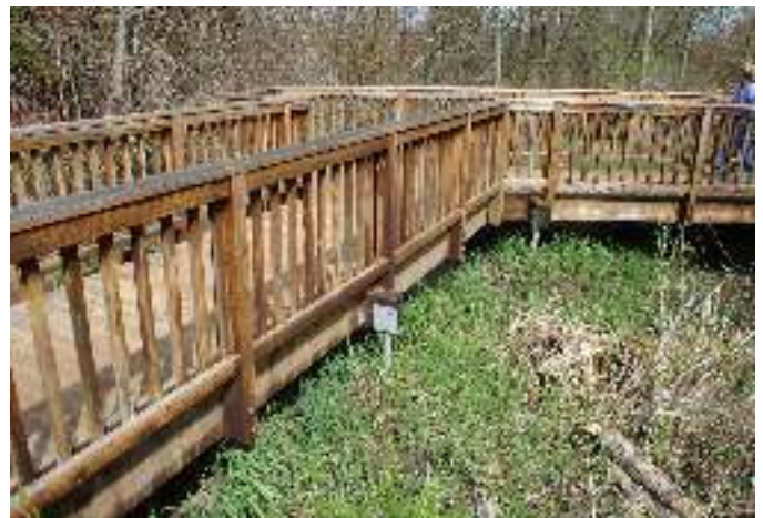
Boardwalk railings assist in keeping trail users away from sensitive areas
