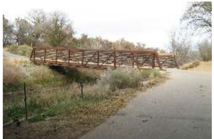
Type 4 Grade-Separated Overcrossing
