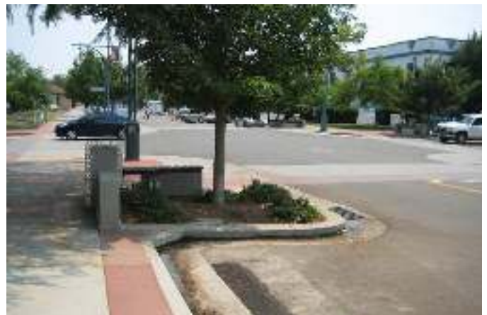
A curb extension can effectively narrow the width of the roadway.
