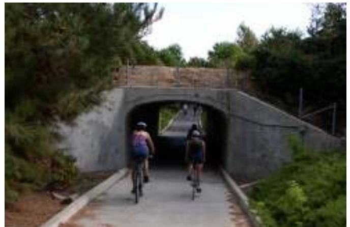
Type 4 Grade-Separated Undercrossing
