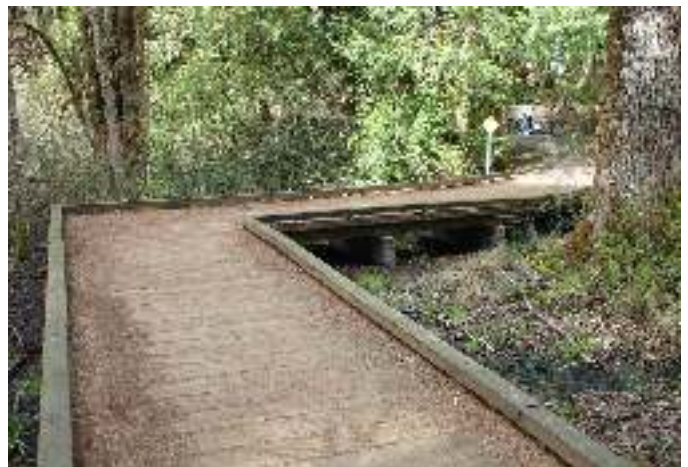
Elevated trail segment allows trail connectivity along a sensitive slope
