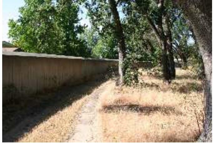
Flood wall adjacent to trail and residences
