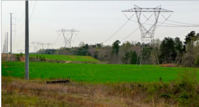
Utility Corridor in east Lincoln County
