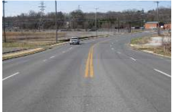
Typical configuration of area roadway
