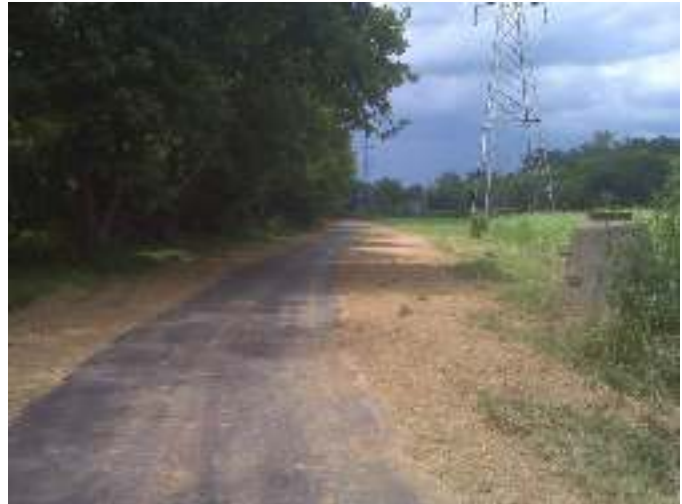
Statesville Greenway Under Construction (Source: City of Statesville Recreation and Parks Department)
