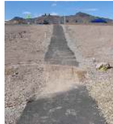
Debris on an asphalt paved trail due to improper drainage design
