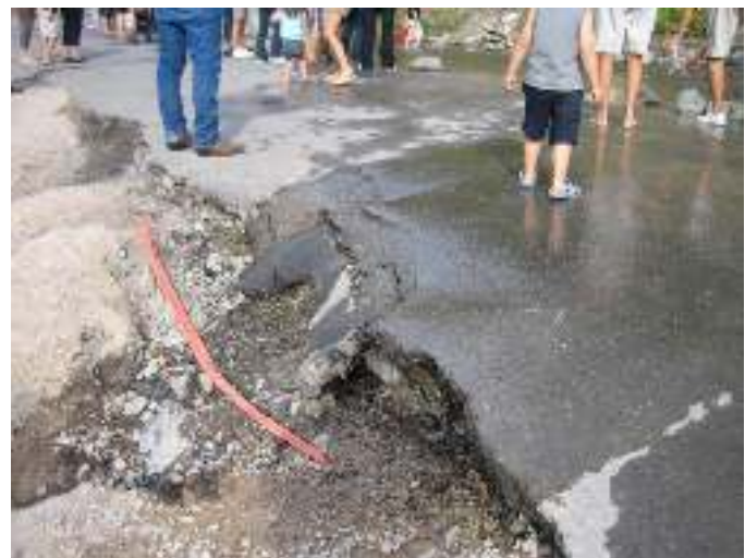
Water erosion undercuts an asphalt trail surface, posing a safety issue for trail users and costly maintenance repairs.
