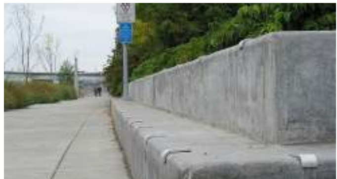
Retaining wall doubles as seating
