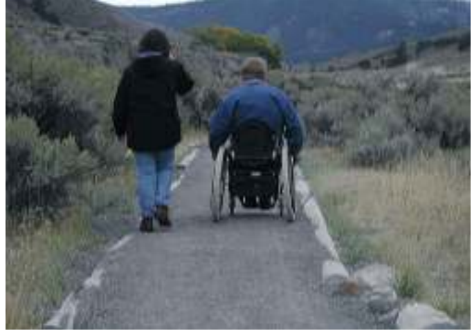
Non-paved surfaces can meet the needs of users with disabilities when properly constructed
