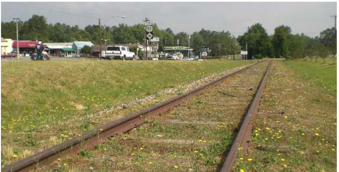
Rail Corridor in Troutman (Source: Centralina Council of Governments)
