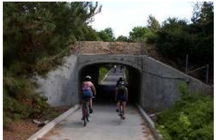
Type 4 Grade-Separated Undercrossing
