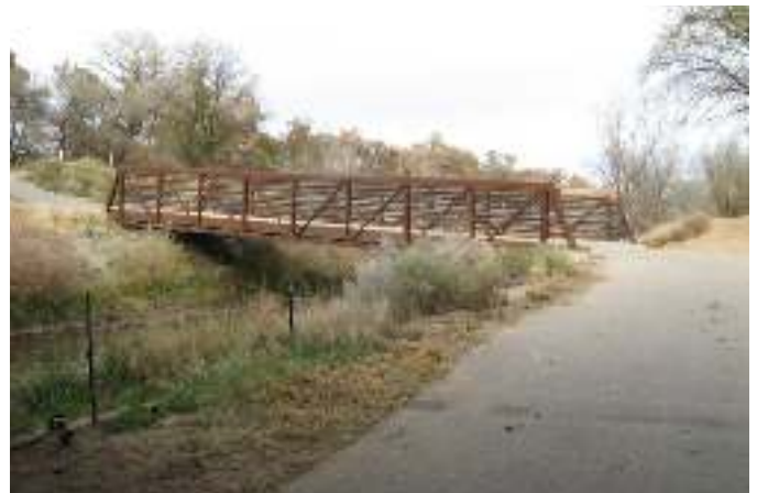
Type 4 Grade-Separated Overcrossing
