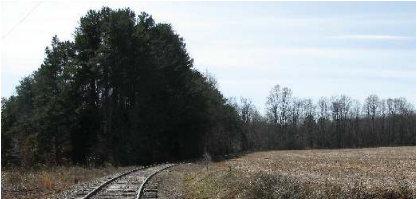
Inactive rail corridor between Newton and Maiden
