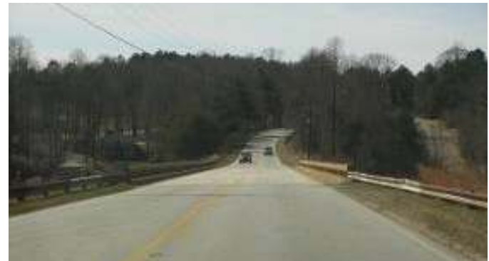
Bridged Crossing at Slanting Bridge Road
