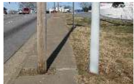
Utility Conflict in sidewalk
