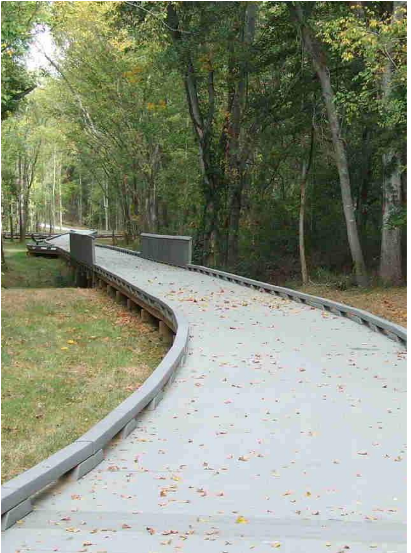
Walkway at Phar Mill Road Park
